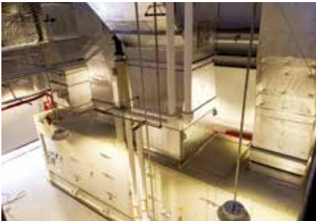
Natural gas turbine with insulated ductwork.
