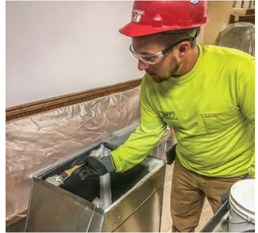
Sheet Metal Foreman Jerry Brown, seals the installation
