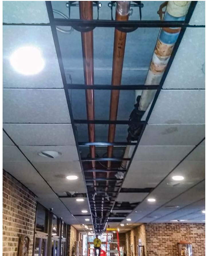
After: New copper piping installed in the ceiling.
