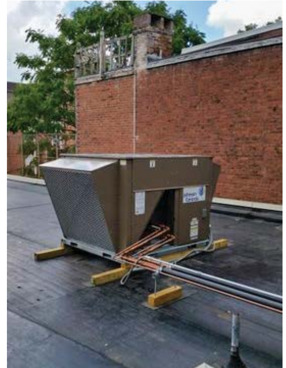
Roof-mounted condenser.
