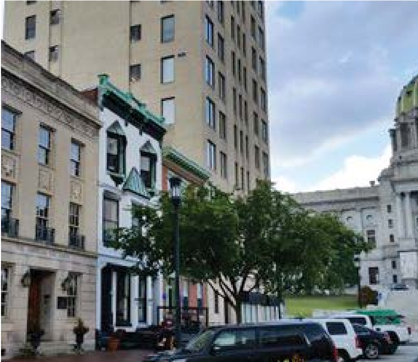
Exterior of Greenlee Partners, LLC in downtown Harrisburg, Pennsylvania.
