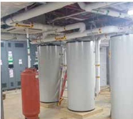
Hot water storage tanks
