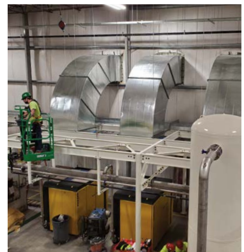
Compressor duct
