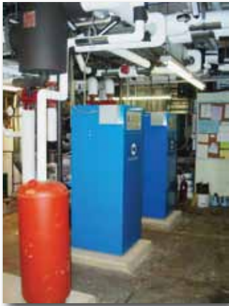
High-efficiency boilers.
