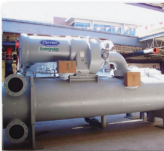
Chiller set in place.
