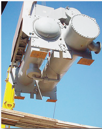
Chiller lowered through the roof access.
