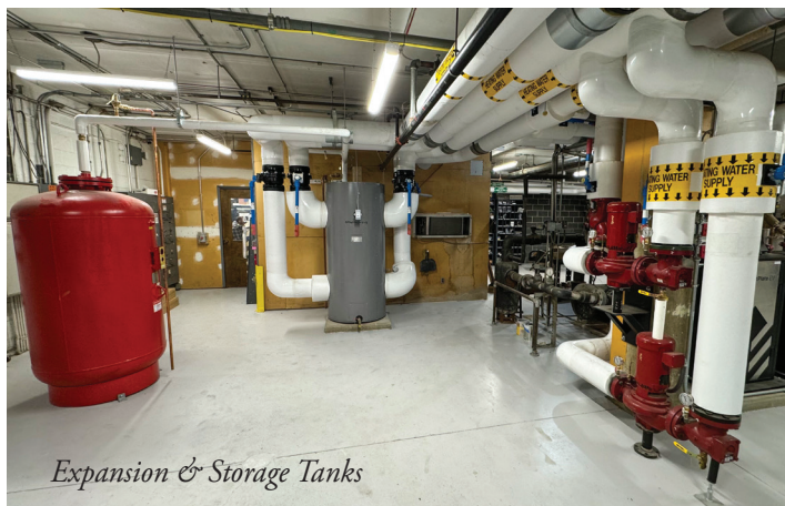
Domestic Hot Water Heat Exchangers
